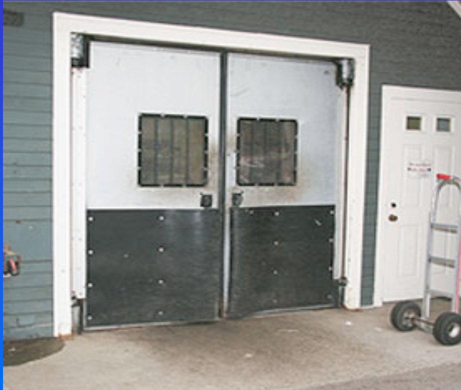
A flexible traffic door and secondary thermal barrier
